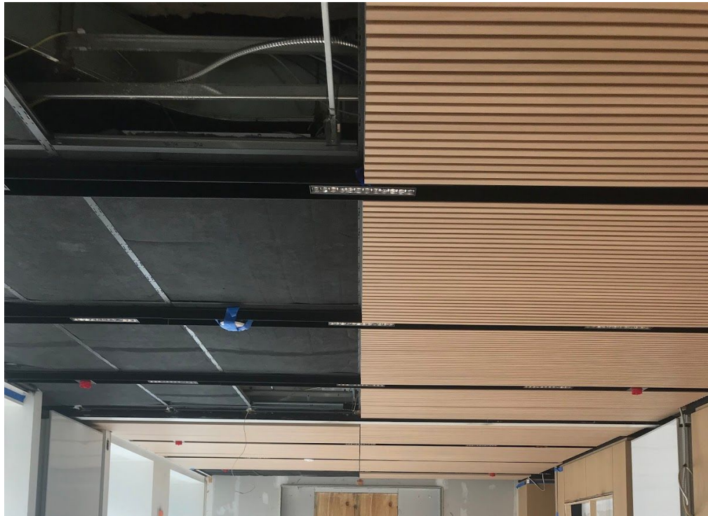
Figure 4.3 - Wood slatted ceiling (right) with absorptive treatment above (left)
