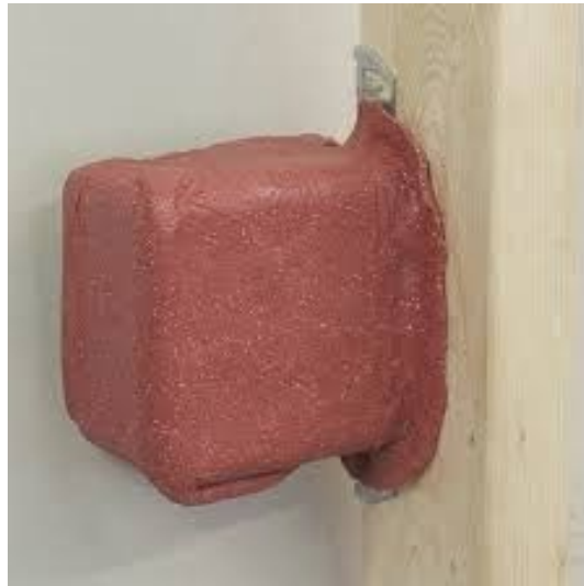
Figure 2.7 - Electrical box with acoustical putty ( Isobacker by Kinetics )
