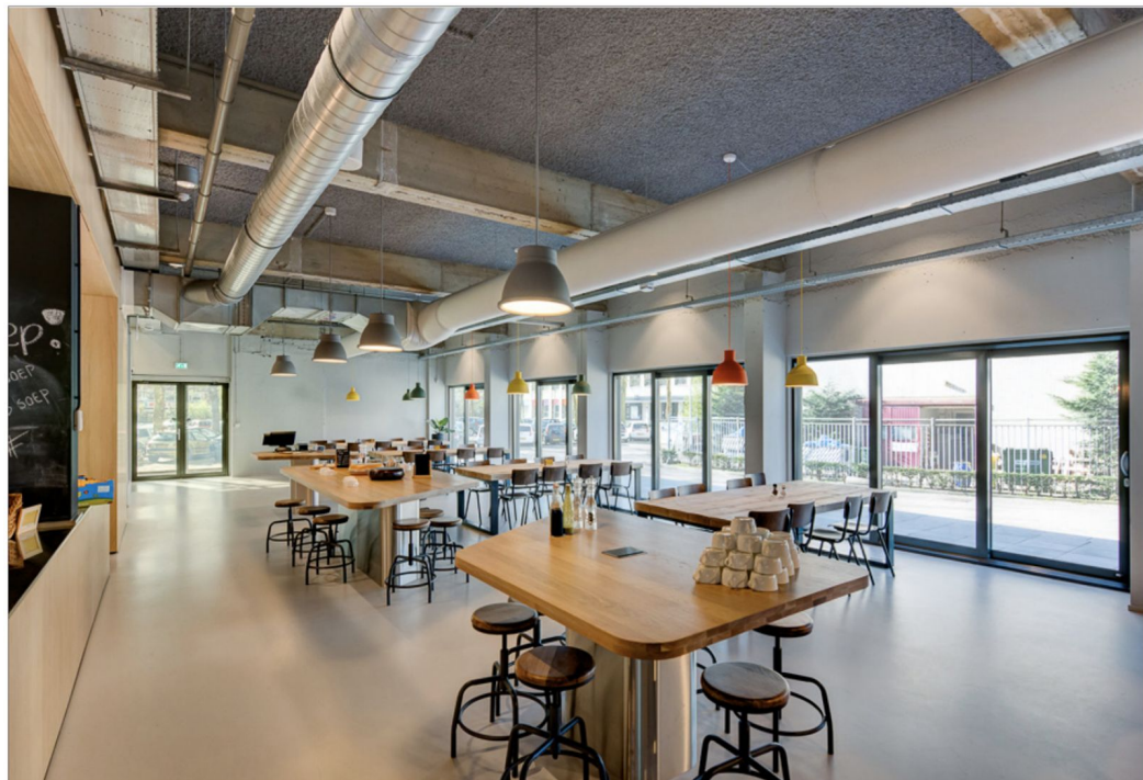
Figure 4.4 - Spray-applied ceiling treatment ( K-13 by International Cellulose )
